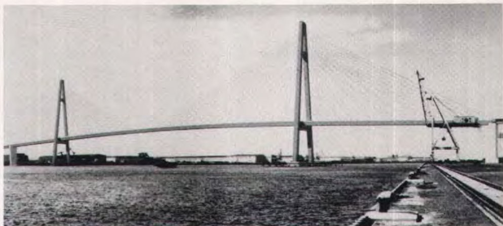
Fig. 3. Nagoya Harbour Bridge, Japan.
