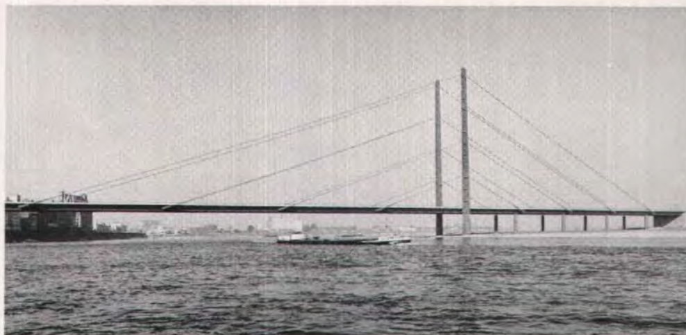
Fig. 16. The slender free standing towers of Kniebrücke in Düsseldorf, West Germany.
